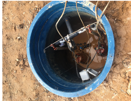
FD- Grinder Pump Final Testing
